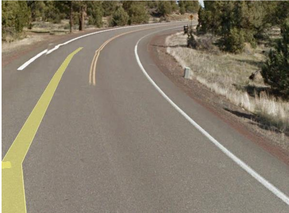
Cline Falls Road: pre chip seal • 12' travel lanes, 3' shoulder
