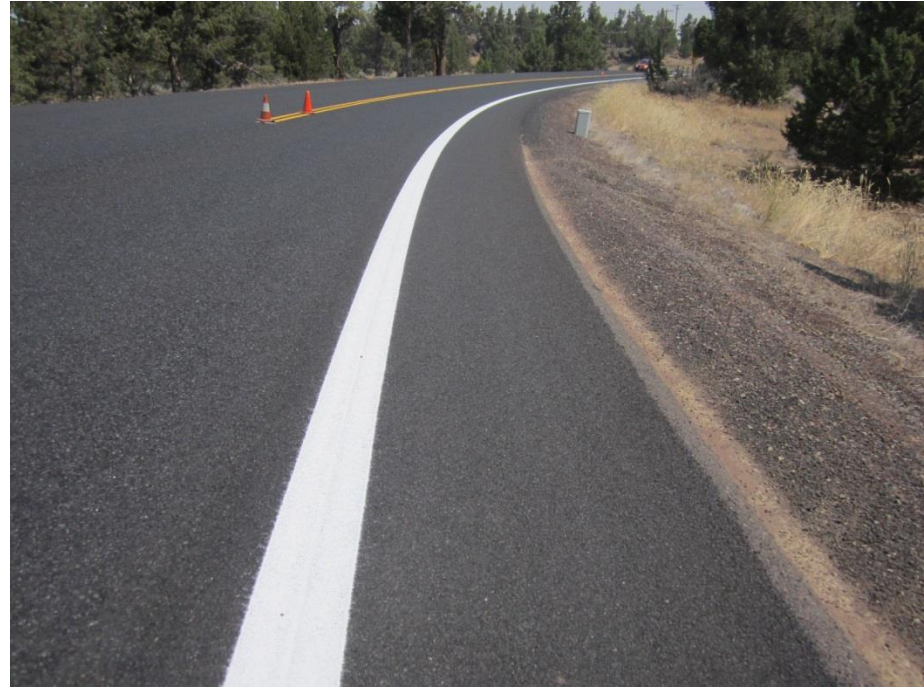
Cline Falls Road: post chip seal • 3/8" chip travel lane • 1/4" chip bike lane • 11' travel lanes, 4' bike lane
