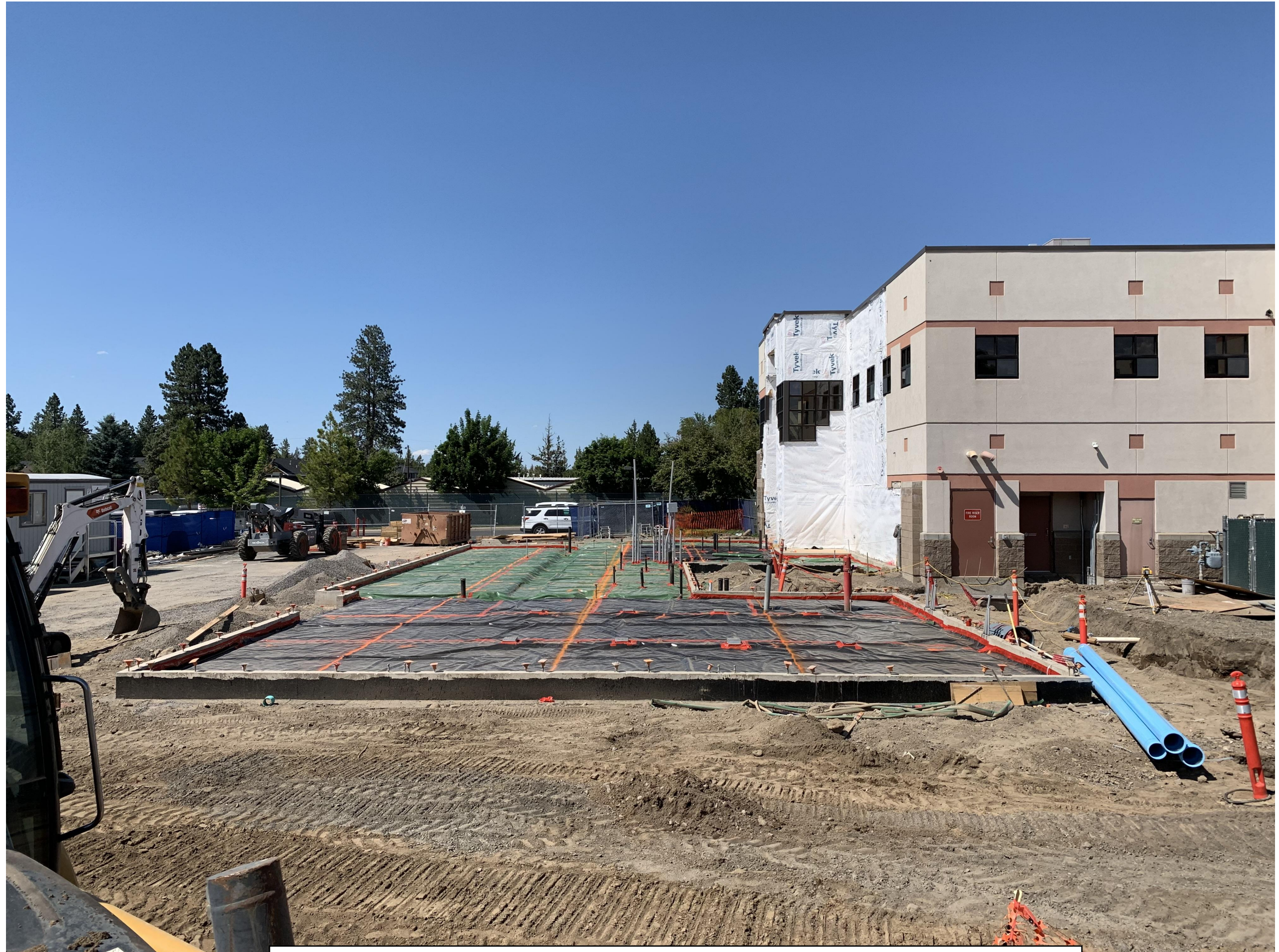
Building Pad - Vapor Barrier Installed, Ready for Reinforcement
