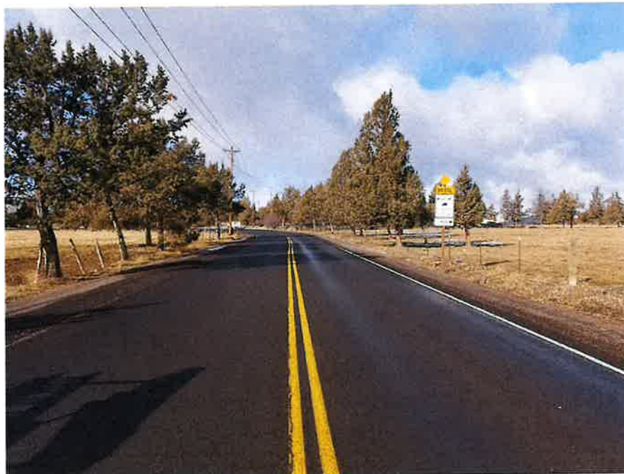
Advanced Warning Viewing West
