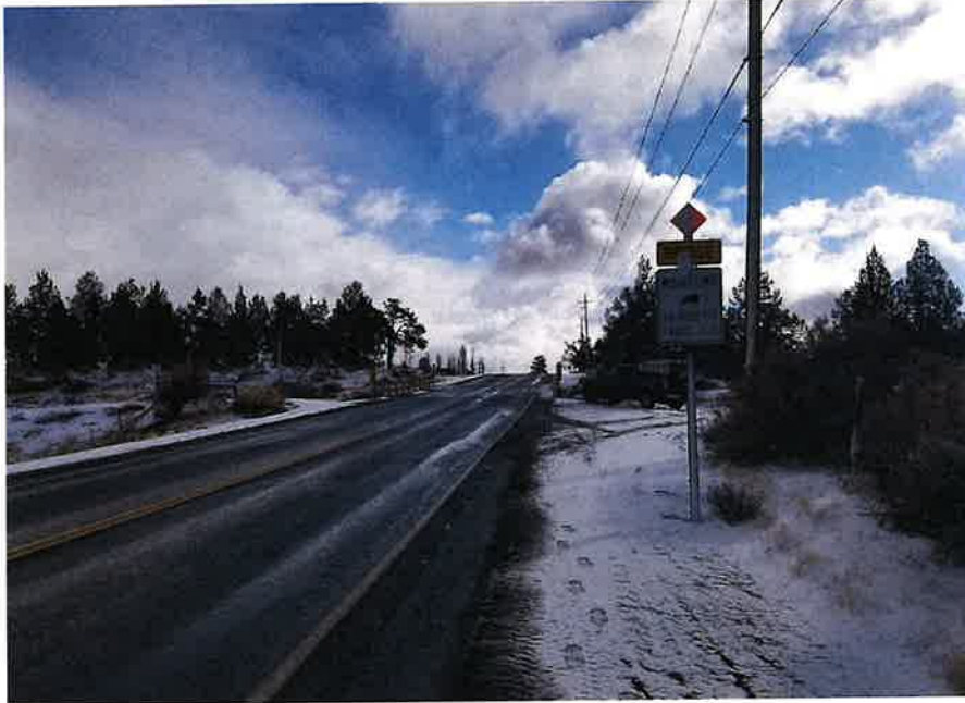
Load Posting Viewing East
