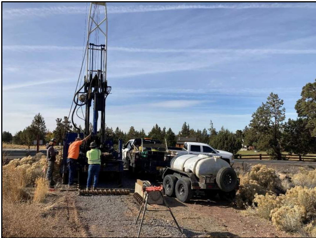
Geotechnical borings performed with truck-mounted CME 850 drilling rig.
