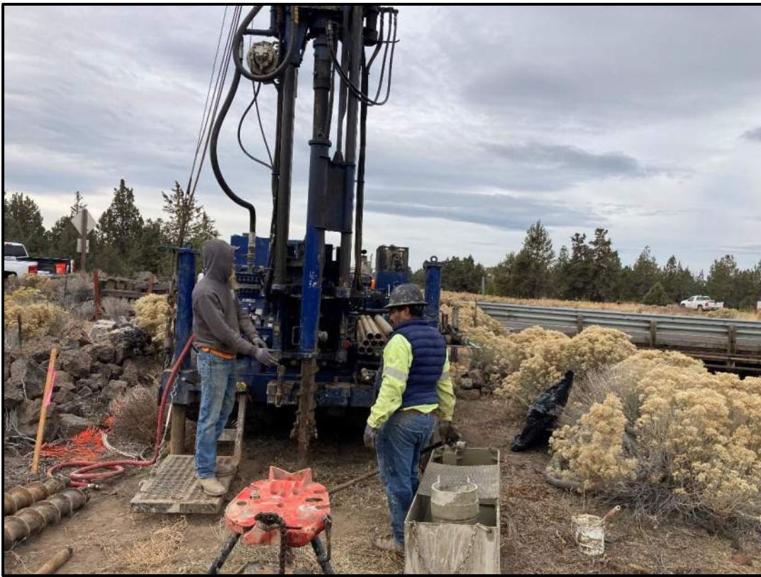
Drilling methods included hollow stem auger and HQ-wireline coring.
