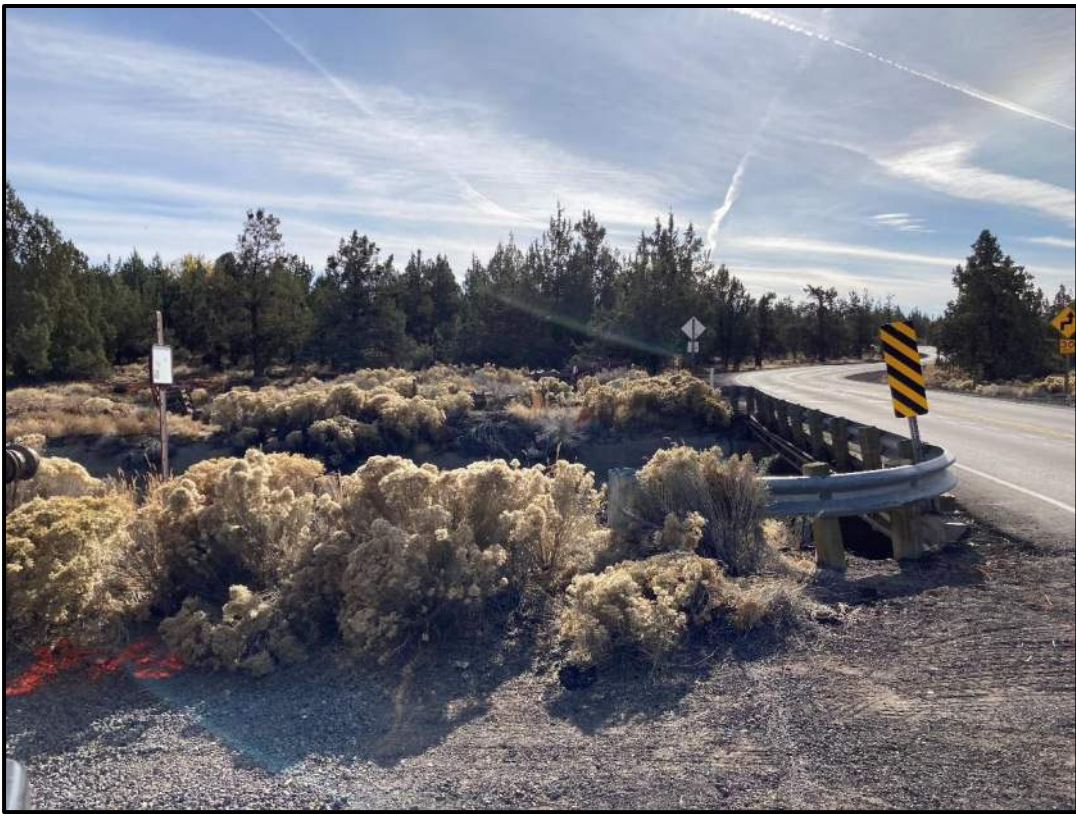
Existing conditions during exploration.
