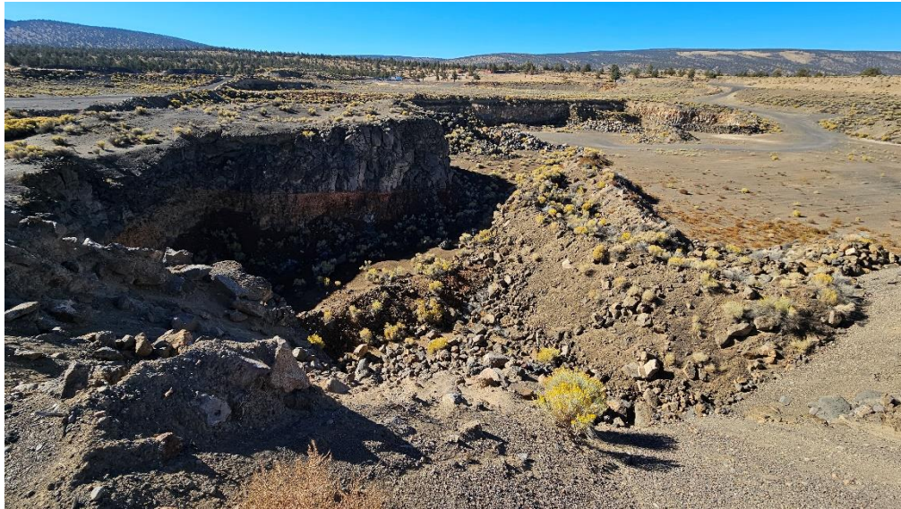
Photo 5. The rock quarry pit in the northwest portion of the Site, as seen from the north. Exposed in this portion is approximately 30 feet of basalt overlying interflow sediment.
